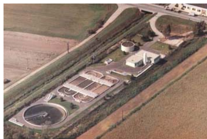
WTP & Other Corrosive Conditions
